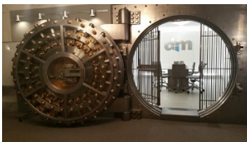
Figure 3.5.1: The hinge on a door such as the one shown above will only allow for rotation along the axis of the hinge. Since this corresponds to moments along the axis of the hinge, it may be useful to specifically calculate the moment a force exerts about the axis of the hinge. Public Domain image, no author listed.
