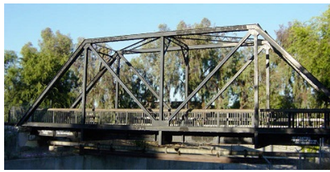
Figure 5.1.2: This bridge is an example of a truss. It consists of a number of members connected at only two points (the ends of the beams). Public domain image by Leonard G.
